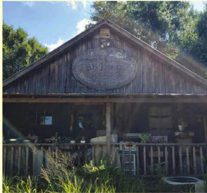
This cracker house replica, built for a movie, now is part of the landscape at the preserve.
